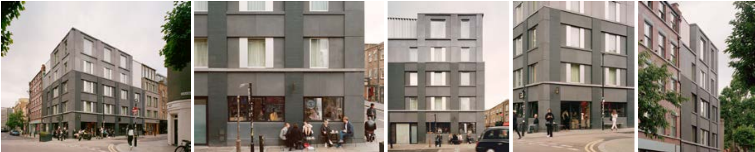
Redchurch Corner, 31/34 Architects, Shoreditch, London
