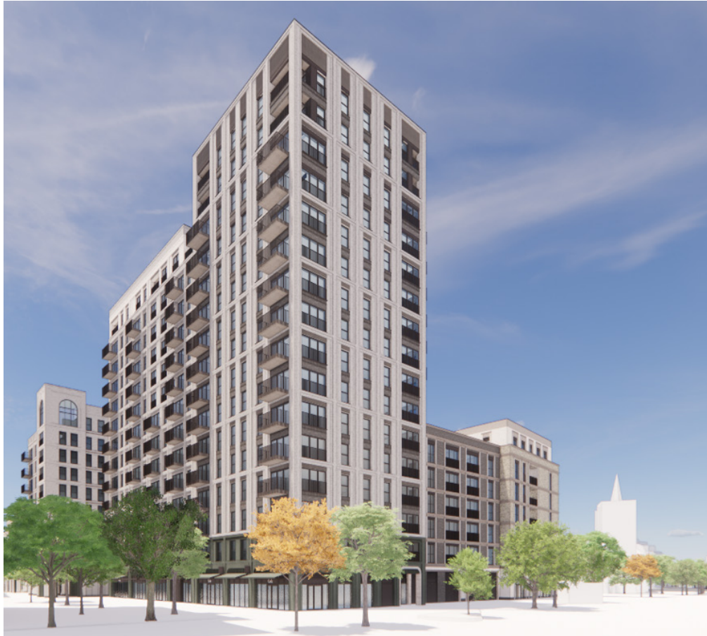
Image: View of Building/Block A2 looking south west
