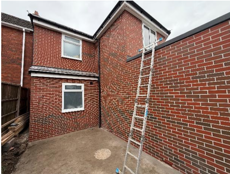
Fig 3 Brick slips applied
