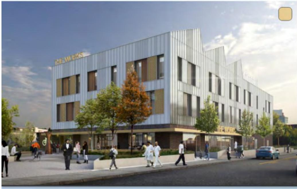
8.3 The dimensions of the building are a foot print of 21m (W) by 45m (L) with an overall height of 16.2m to the saw tooth apex reducing to 13.2m to the flat roof. The concept of the building is a grid shape of rooms which would be 7m by 7.5 metres (see ground floor plan arrangement below).
