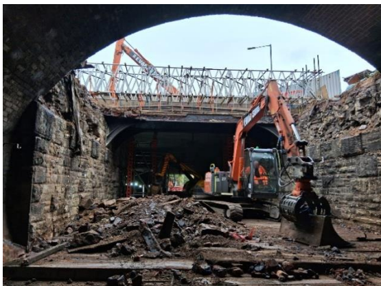
Whitefield Tunnel Renewal during the demolition work
