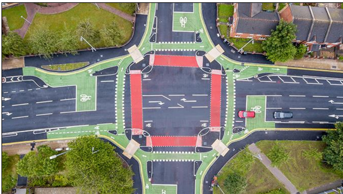
Example CYCLOPs delivered at Royce Rd / Chorlton Rd junction
