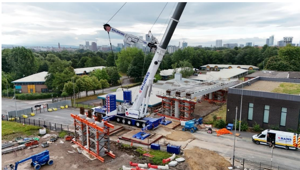
Salford Rise: Bridge over Frederick Road being moved into place
