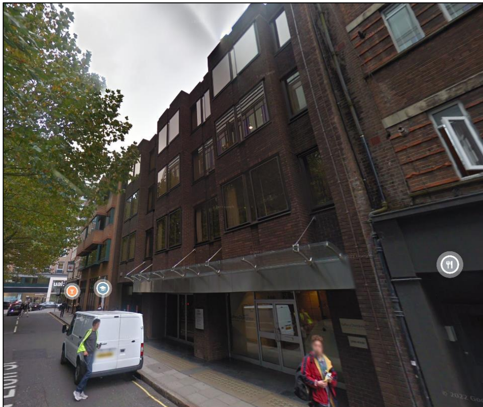
Figure 2: Streetview of the application site
