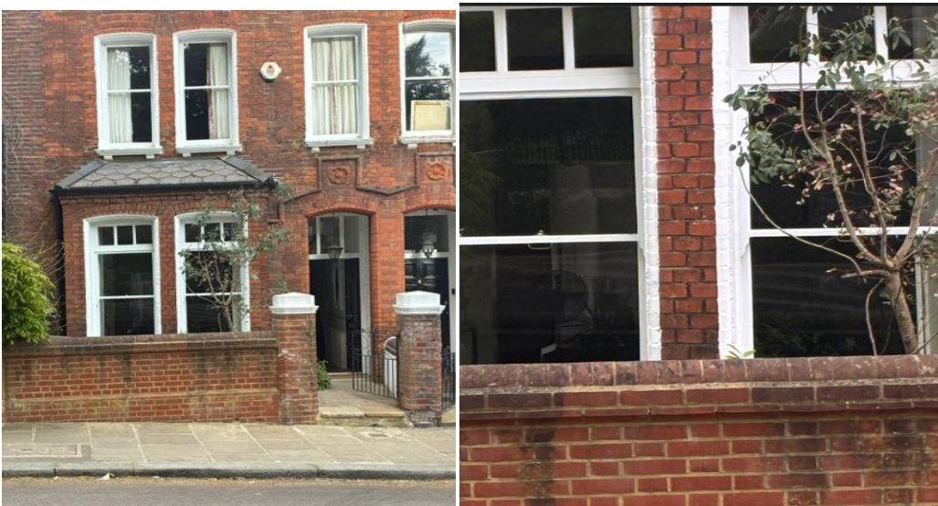
Images 7 and 8: View drinkers would have from new kerb seating- steps directly into sitting room & first floor of 6 Well Walk
