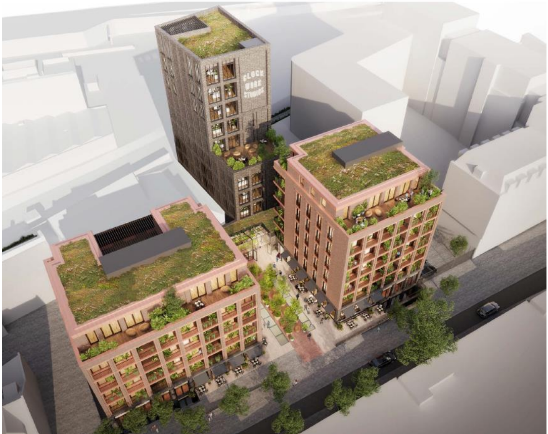
Figure 53 - Granted scheme at Asher House (Clockwork Factory)
