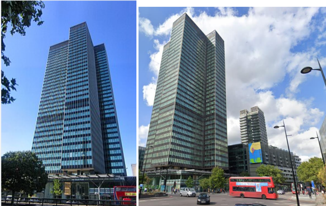
Figure 2 – Images of the existing Euston Tower
