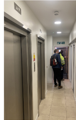
Narrow lift lobbies (not Part M compliant)
