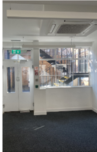
Level 1 fire escape
