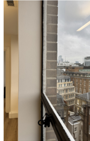
Existing single-glazed windows
