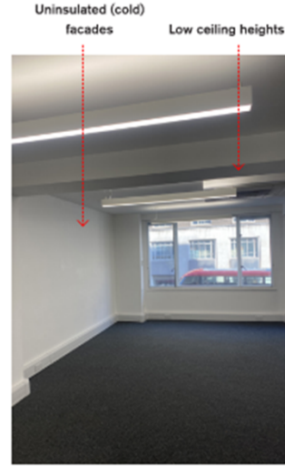
Typical office space
