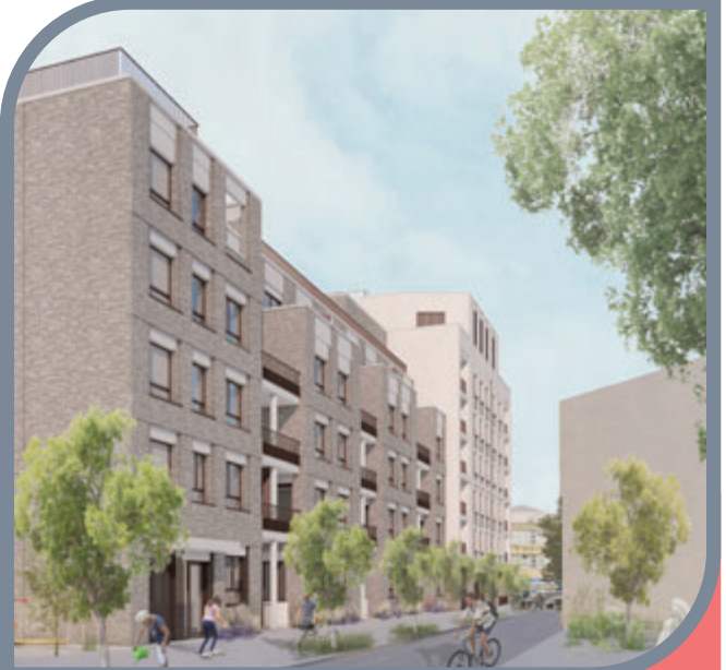
Planning secured for West Kentish Town
