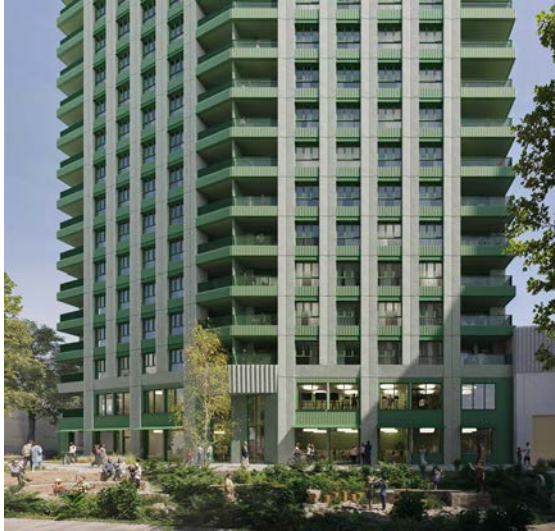
Figure 35 - The south-west elevation of B1, showing the precast concrete vertical pilasters
