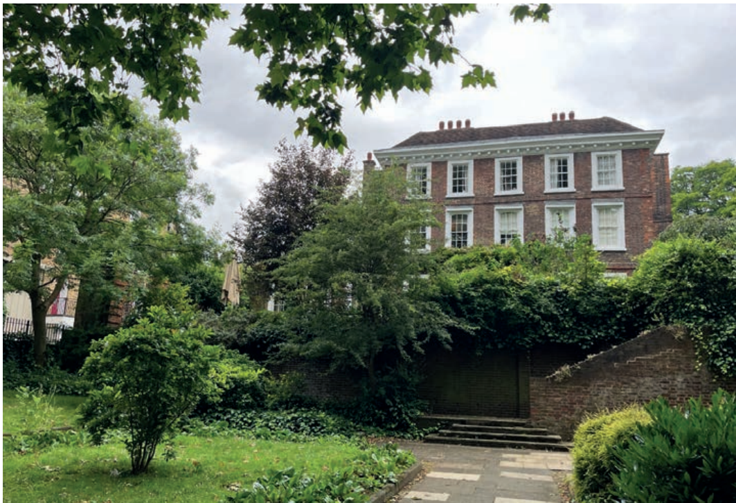
fig. 3.8 Burgh House is a Grade I listed building and an important cultural centre
