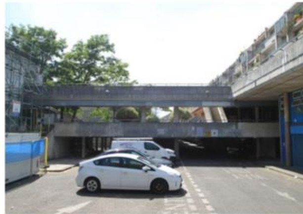
View from level 02 of car park entrance showing existing high level route to Block A. Casing to be replaced by smaller/higher pipework
