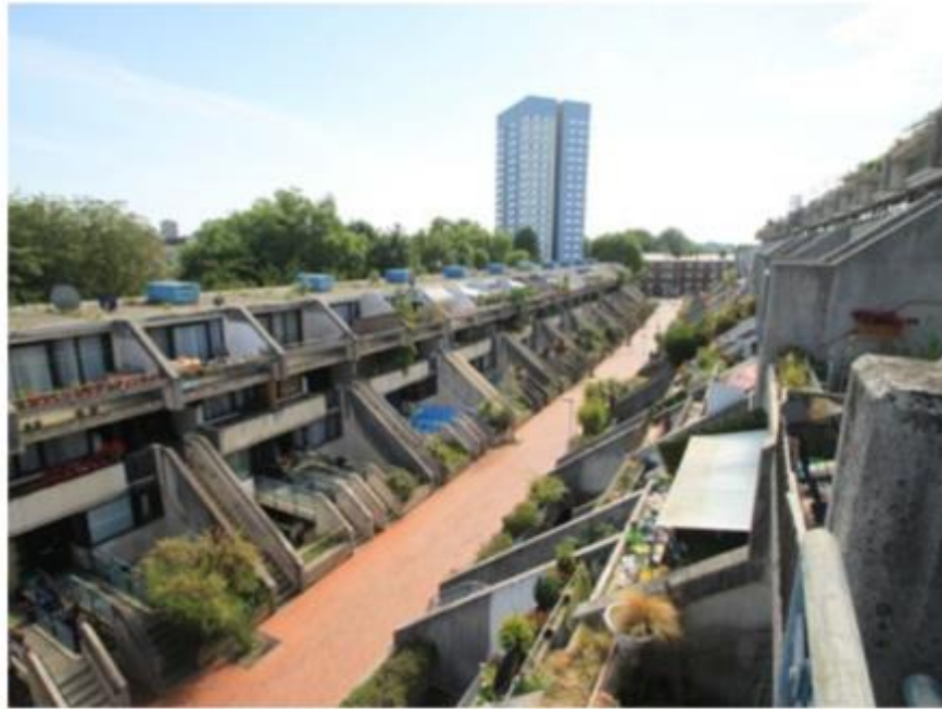
View South-Wet to block B from Block A Staircase
