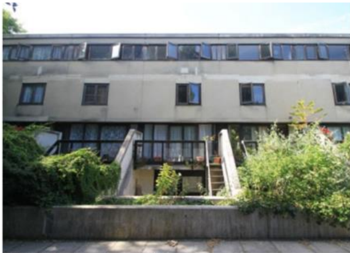
Block B South Elevation, seen from Langtry Walk
