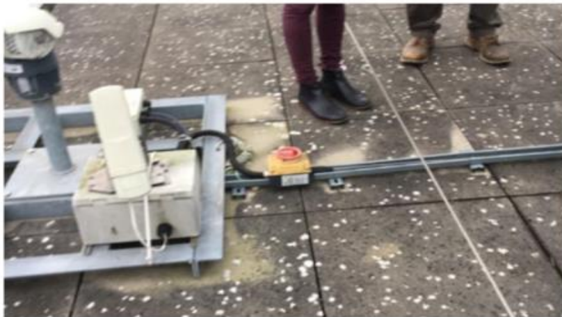
Typical bracing currently used elsewhere on Block B roof
