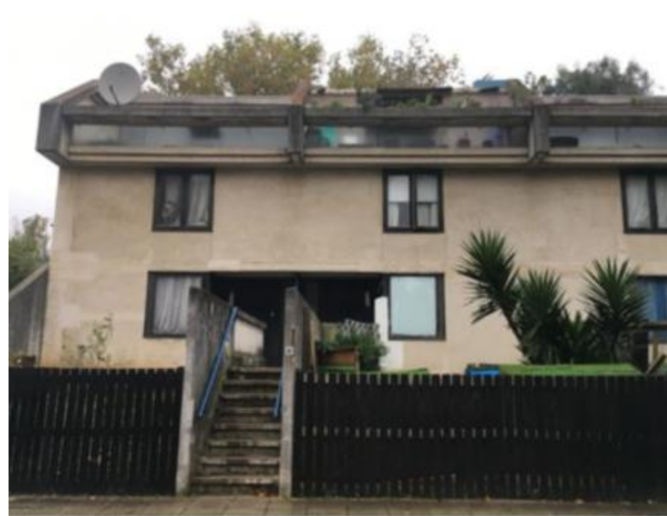
Block C from Boundary road (South elevation)
