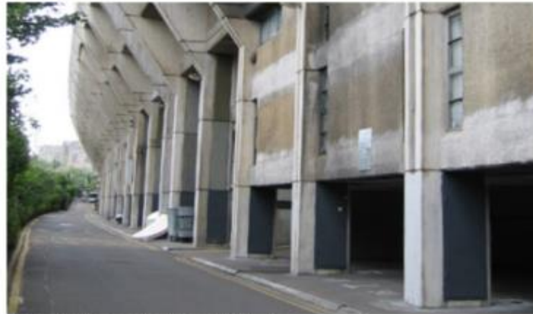
1. Existing Block A ground condition - North Elevation
