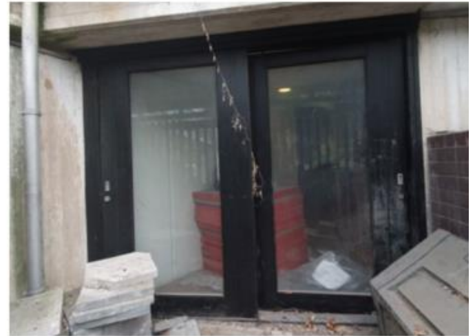
2. View of Existing Doors from Bin Store.
