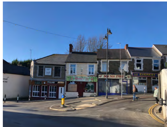
Level changes and wide road at Pentwyn Rd junction
